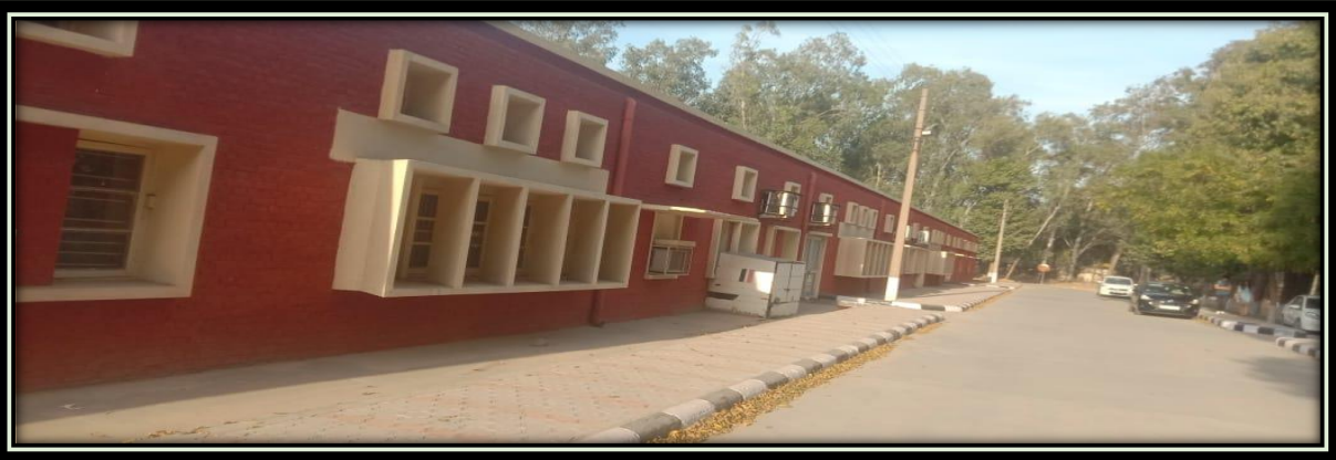
Fig.3 Roof top rainwater harvesting pipelines for tapping rainwater.
