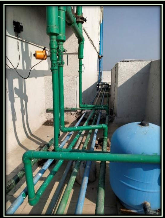
Fig.5 STP and dual plumbing for use of STP treated water for meeting flushing requirements in the campus.
